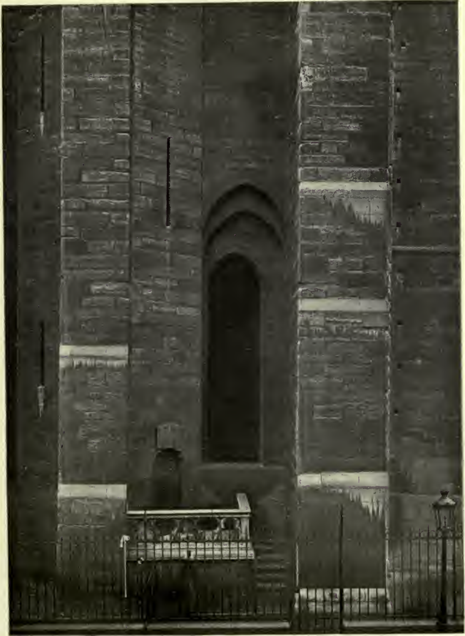
FIG. 4. NOTRE-DAME. DETAIL OF THE EXTERIOR NORTH TOWER CONSTRUCTION. Compare with Fig. 3 and Fig. 5. Note the window ledge as level.
